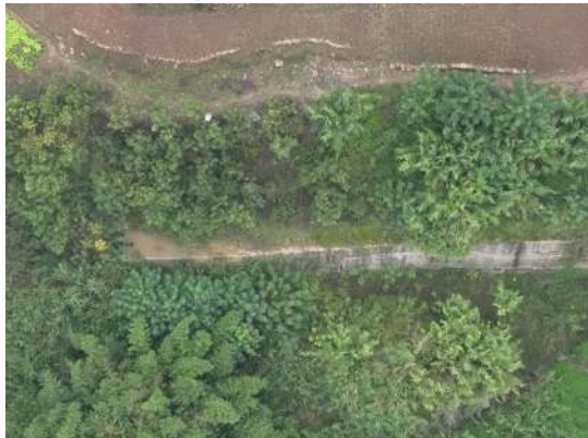
DXP1#弃渣场挡土墙
