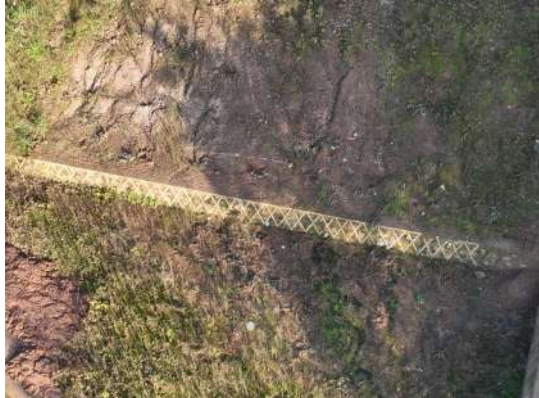
QYJ4#渣场挡土墙
